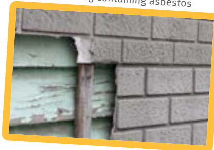
External cladding containing asbestos
