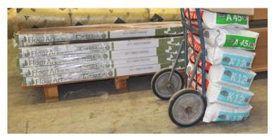
Cartons of tiles should also be handled carefully. Use a trolley to move them around the floor.
