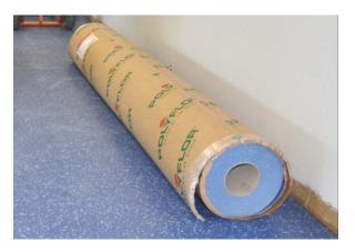
Rolls that are 3 metres wide or more need to be laid down flat on a smooth level surface that supports the entire length of the roll. Make sure there are no objects under the roll that might damage the material or cause pressure marks.
